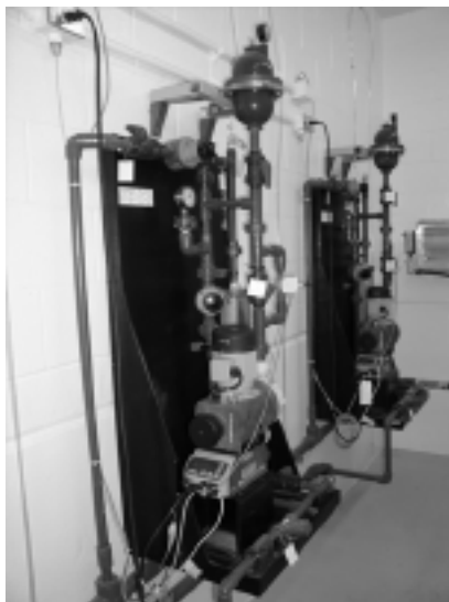
Fort Atkinson uses 3 ProMinent skids for ferric feed.
